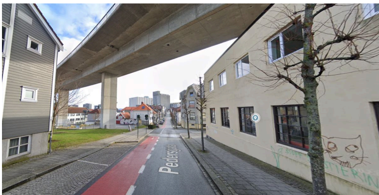
Jammerdalen area with Jammerparken to the left, and Nevlandsbygget to the right.
